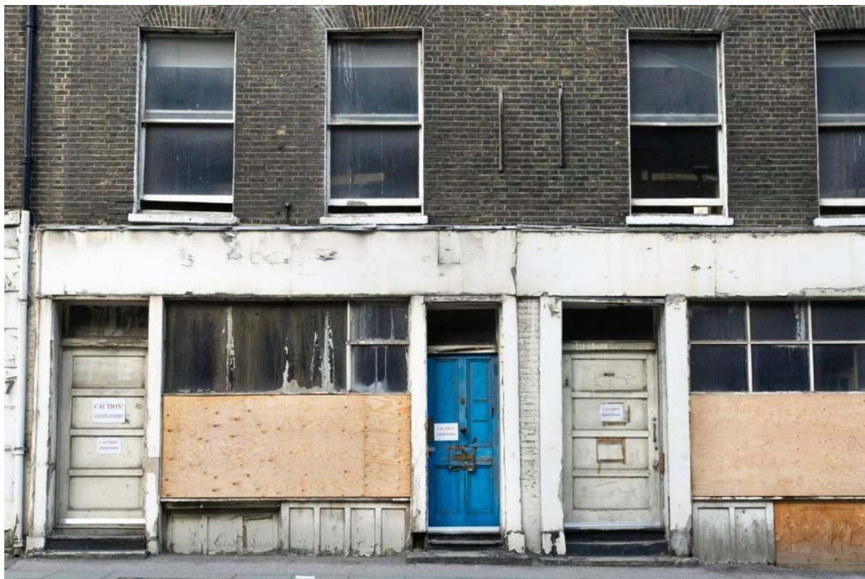
Neglected shopfronts, London, UK. (Photo by BuildPix/Construction Photography/Avalon/Getty Images) GETTY IMAGES
